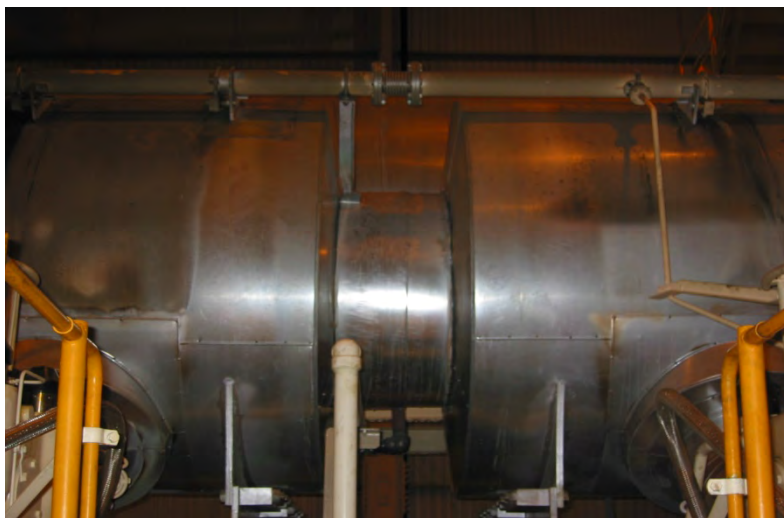
Figure 14. Stress corrosion cracking, in a combustion gases pipe of a thermoelectric station.
